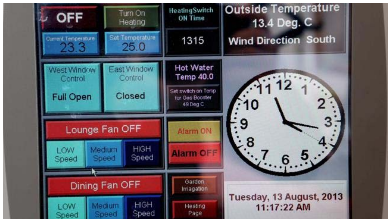
The environment control panel in the Altona North home of Leanne and Jason McHale.
