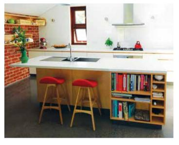
Polished concrete slab floors upstairs and downstairs provide thermal mass in this highly insulated home with a tight building fabric. Double-glazed windows and doors have FSC European Redwood timber frames.
