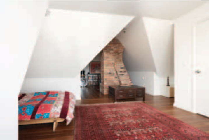
The upstairs addition includes spare bedroom, study "nook" and second bathroom. Nullarbor Timber recycled spotted gum floors were chosen and finished in Livos low VOC oil. The grilles for the heat exchange system are visible to the right of the original chimney (retained as a feature of the room).
