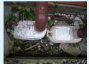
↑ Shown here are both Nylex Greywater Diverta units for the home. Photo by Verity Campbell
